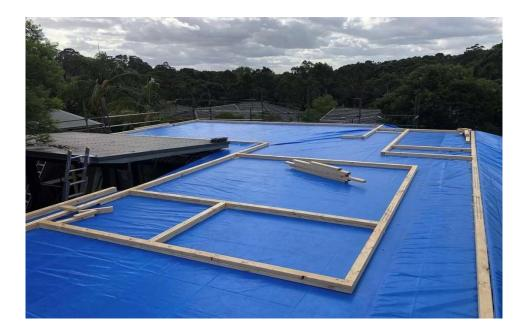
Once down make sure that the BFS is smooth and tight – make sure it is weighted down to ensure it remains in place.
