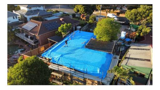
Roll out the BFS allowing at least 1 meter overhang around the outer parameter
