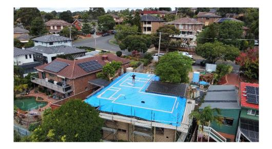
Mark out your framework with a waterproof Black Marker on the Builders Floor Sheet and start laying out the framework
